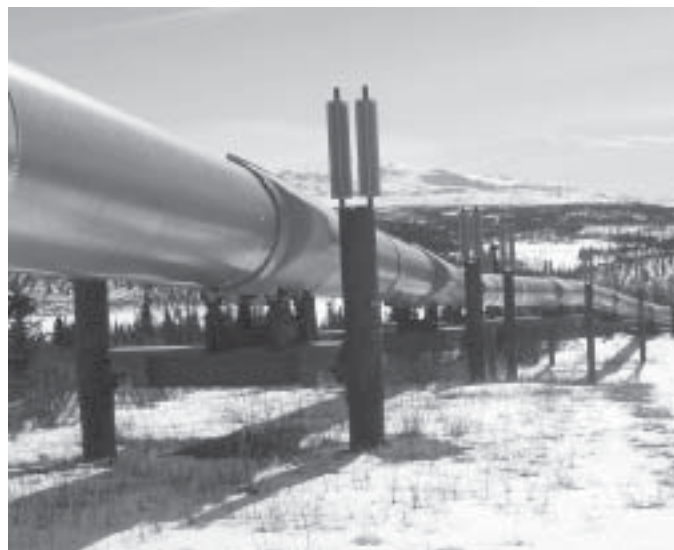
The TransAlaska pipeline, as seen by Russian visitors in April, 2003.
