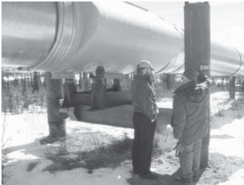
Trip participants get a firsthand look at the TransAlaska pipeline and its special construction meant to survive earthquakes and other threats to its structural integrity.
